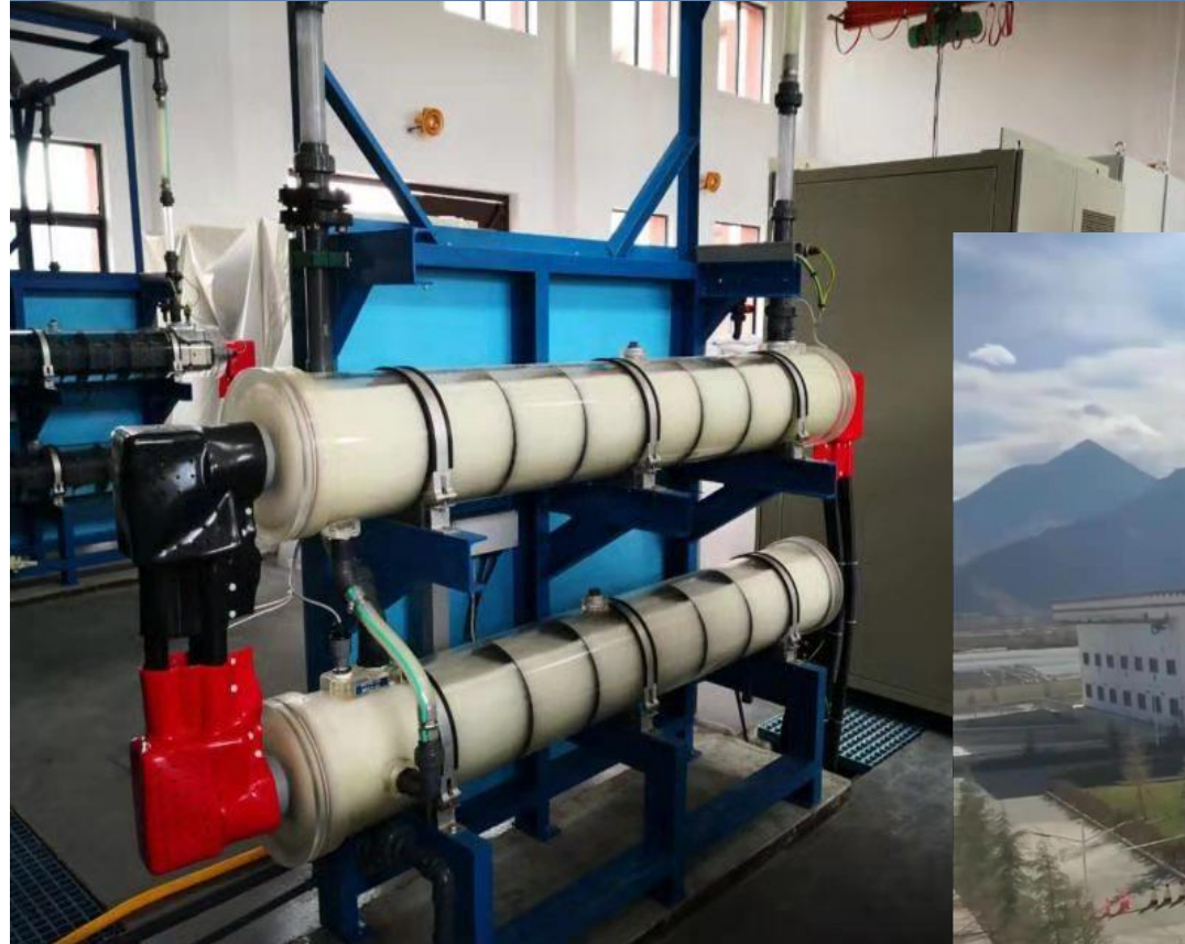
Tibet Lhasa Najin Water Plant Project (Lhasa, China) – 450x4kg/Day Drinking Water Disinfection
